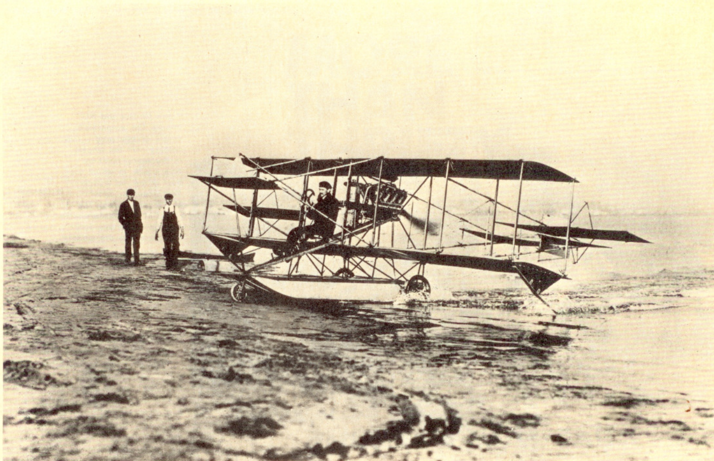
Glenn Curtiss taxis the original Triad amphibian ashore at North Island, San Diego, early in 1911. Note the fixed nosewheel under the bow of the float, and the forward elevator supported by bamboo booms anchored to the wing roots.
